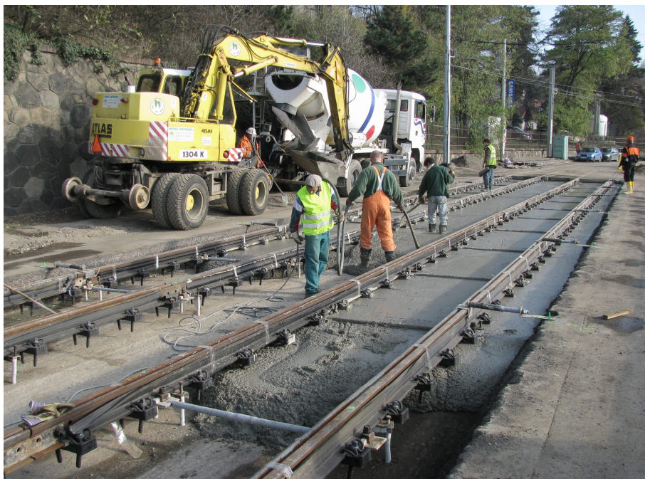
Fig. 2: Concreting the slab under the Vyšehrad in November 2008
