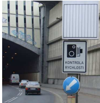
Fig. 5: The warning sign “Measurement of the speed” before the portal of Strahov tunnel
