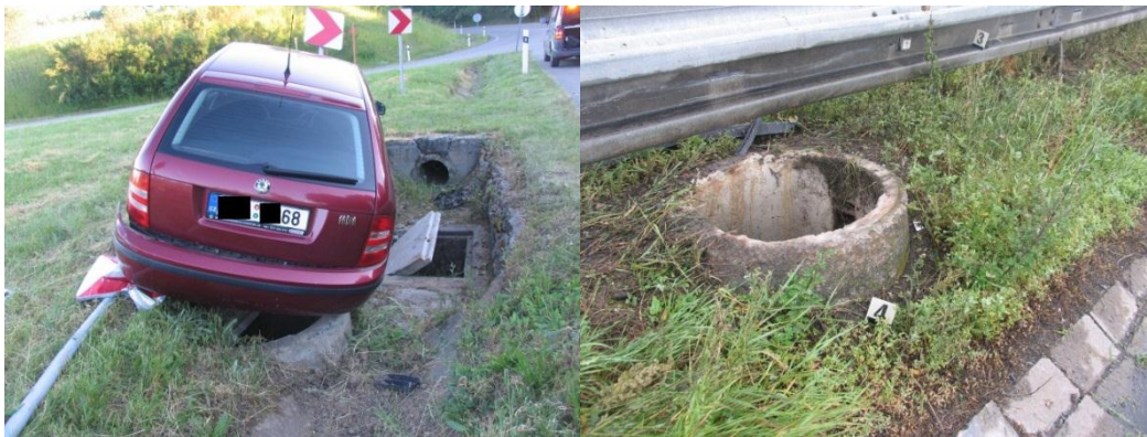
Fig. 13. Problem 6 – detail of concrete canalization shaft
