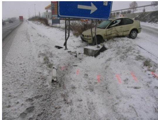
Fig. 9. High risk location 2 – concrete bases of traffic sign above the terrain
