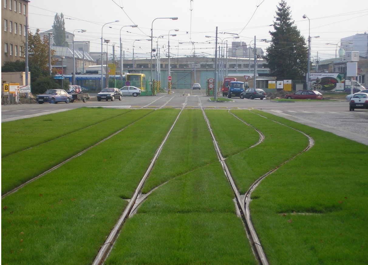
Fig. 6: Track with an artificial irrigation system – Plzeň, the Slovanská alej Street
