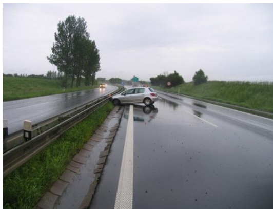
Fig. 11. High risk location 4 – detail of condition of the road surface with crashed vehicle
